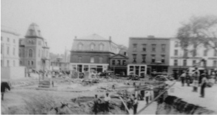
Digging the foundation of City Hall, where Burlington Town Hall and Chittenden County Courthouse #3 used to be. (Notice Courthouse #4 and #5 in the background).
